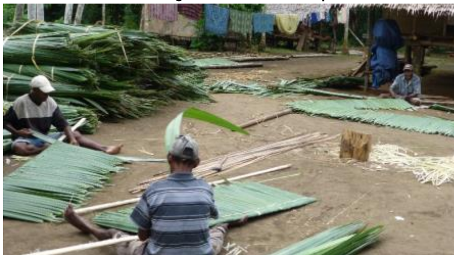
Plate 9.19 – Men Making Roof Thatch From Nipa Palm at Avavu
