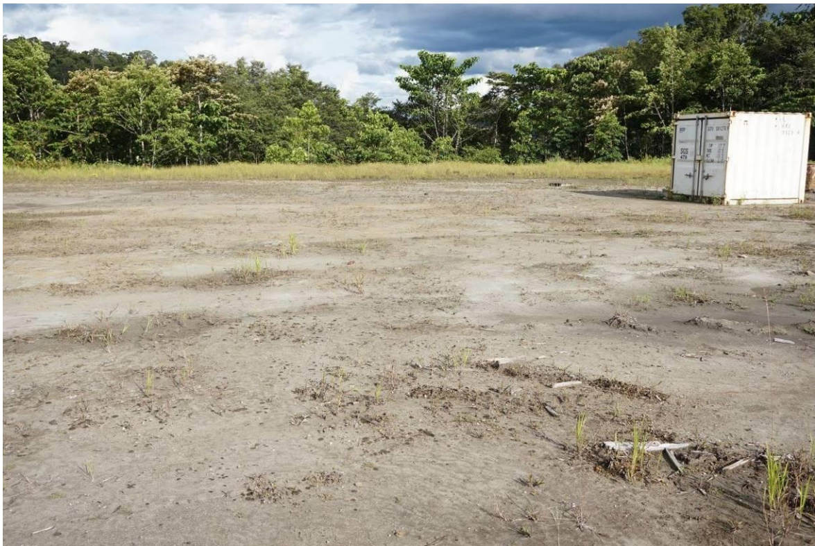
Plate 8-9 Bare hardpack wellpad surface
