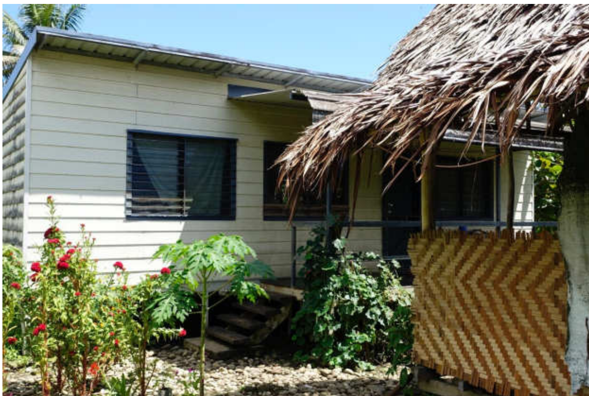
CHW house at Wabo Station.
