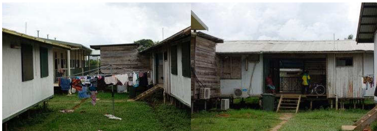
Plate 22. Kerema Health Center Inpatient Facilities
