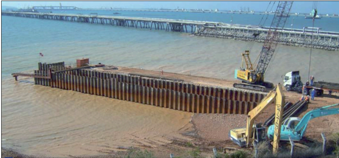
Plate 1 – Example of Shoreline and Nearshore Pipeline Trenching Works
