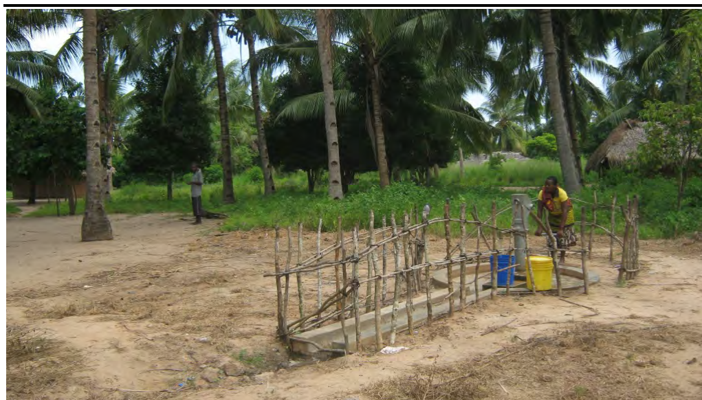
Figure 8.10 Typical Community Borehole Equipped with Handpump (Senga Village)
