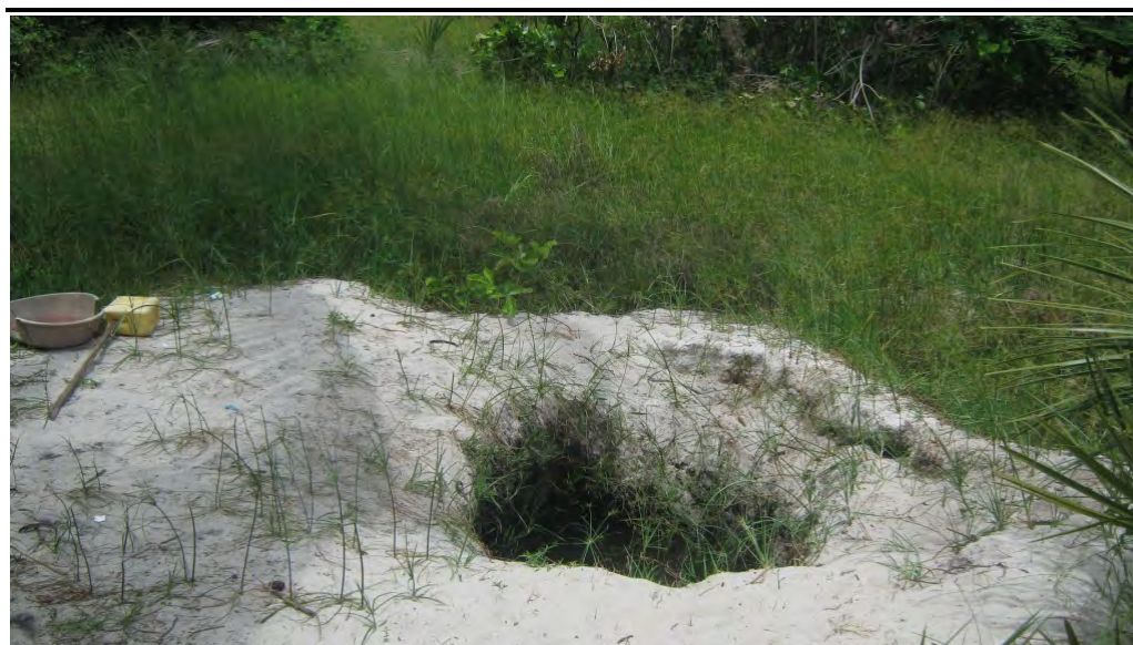
Figure 8.11 Typical Hand-dug Well Used for Community Water Supply
