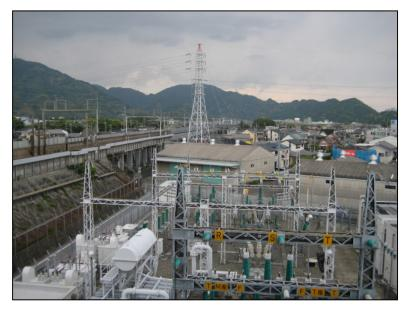
Figure 19: Photo of Typical Traction Power Substation on Tokaido Shinkansen in Developed Area
