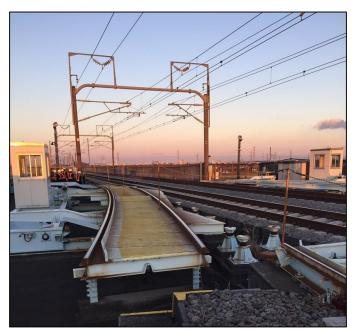
Figure 33: Mechanical Siding-off Temporary Track Connection
