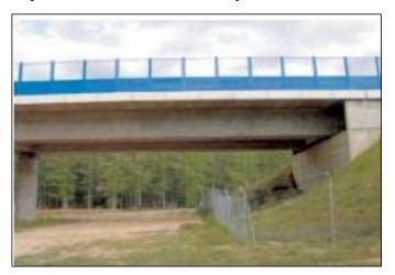
Figure 44: Example of security fence along transition from embankment to viaduct (Courtesy of the Ministry of the Environmental of Spain). Note that the area beneath the viaduct can be traversed freely by wildlife or cattle.
