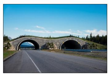
Figure 47: Example of a wildlife overpass crossing of highway.
