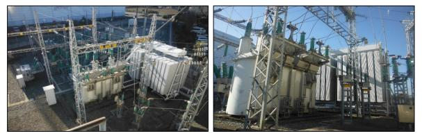
Figure 17: Typical Traction Power Transformers
