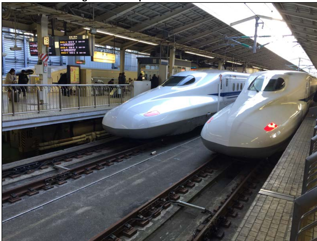
Figure 2-10: Japanese Station Platform
