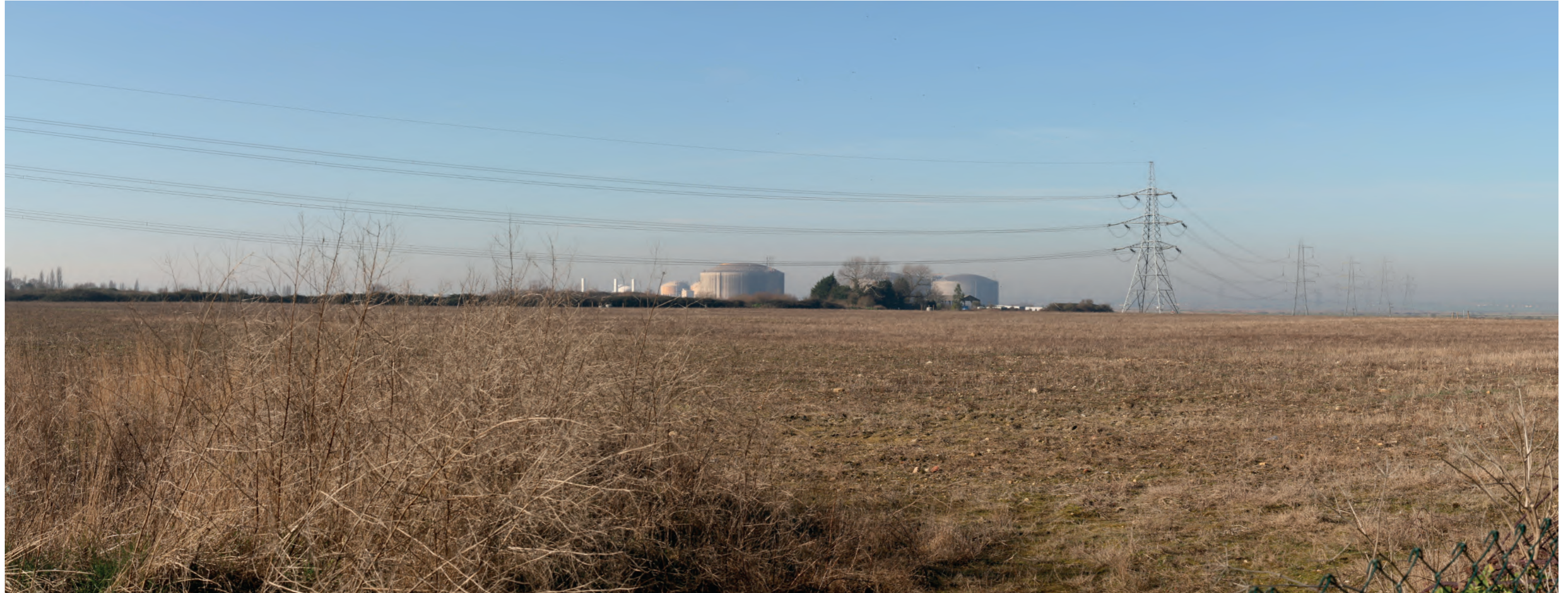
Figure: 5.9a Viewpoint 2 - West Lane Existing View
