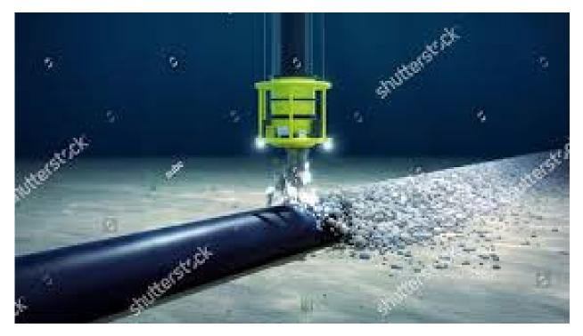
The placement of specifically graded rock on a surface laid cable to protect against external threats such as fishing and dragged non holding anchors, is a well-established protection method in the North Sea area.
