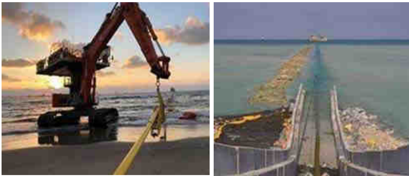
Figure 6-13: Examples of shore approaches by float-out method
