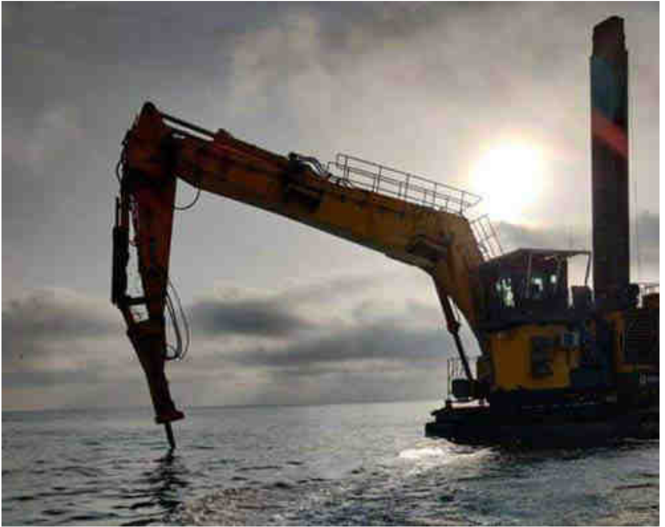
Figure 4-77: BHD fitted with hydraulic hammer
