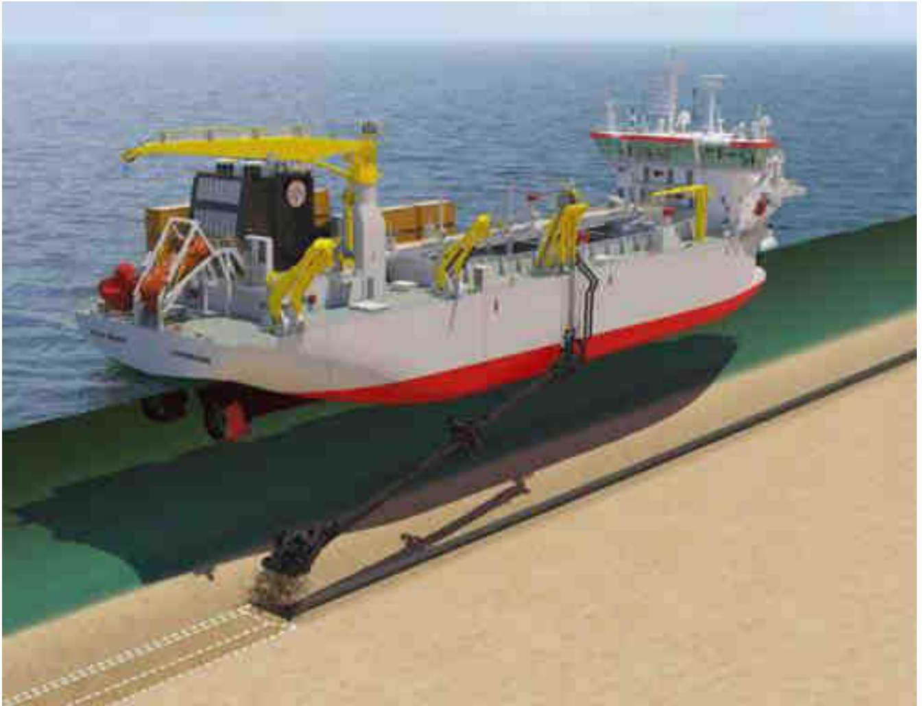
Figure 4-82: TSHD backfilling through suction pipe
