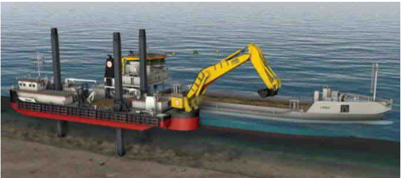
Figure 4-76: Clean up dredging
