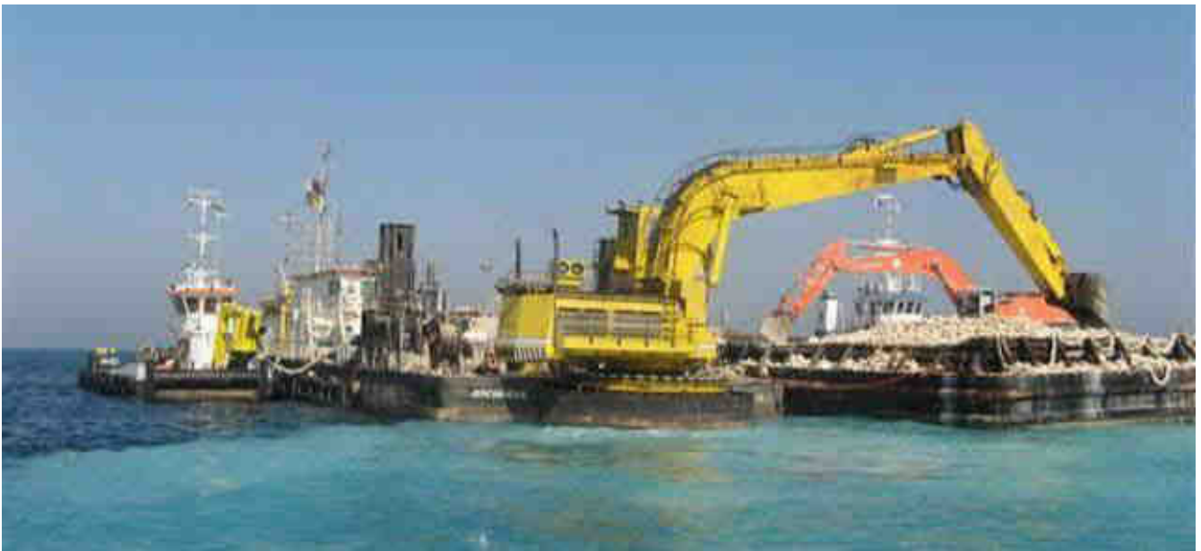
Figure 4-81: HD 'Jerommeke' bac filling material from a pontoon
