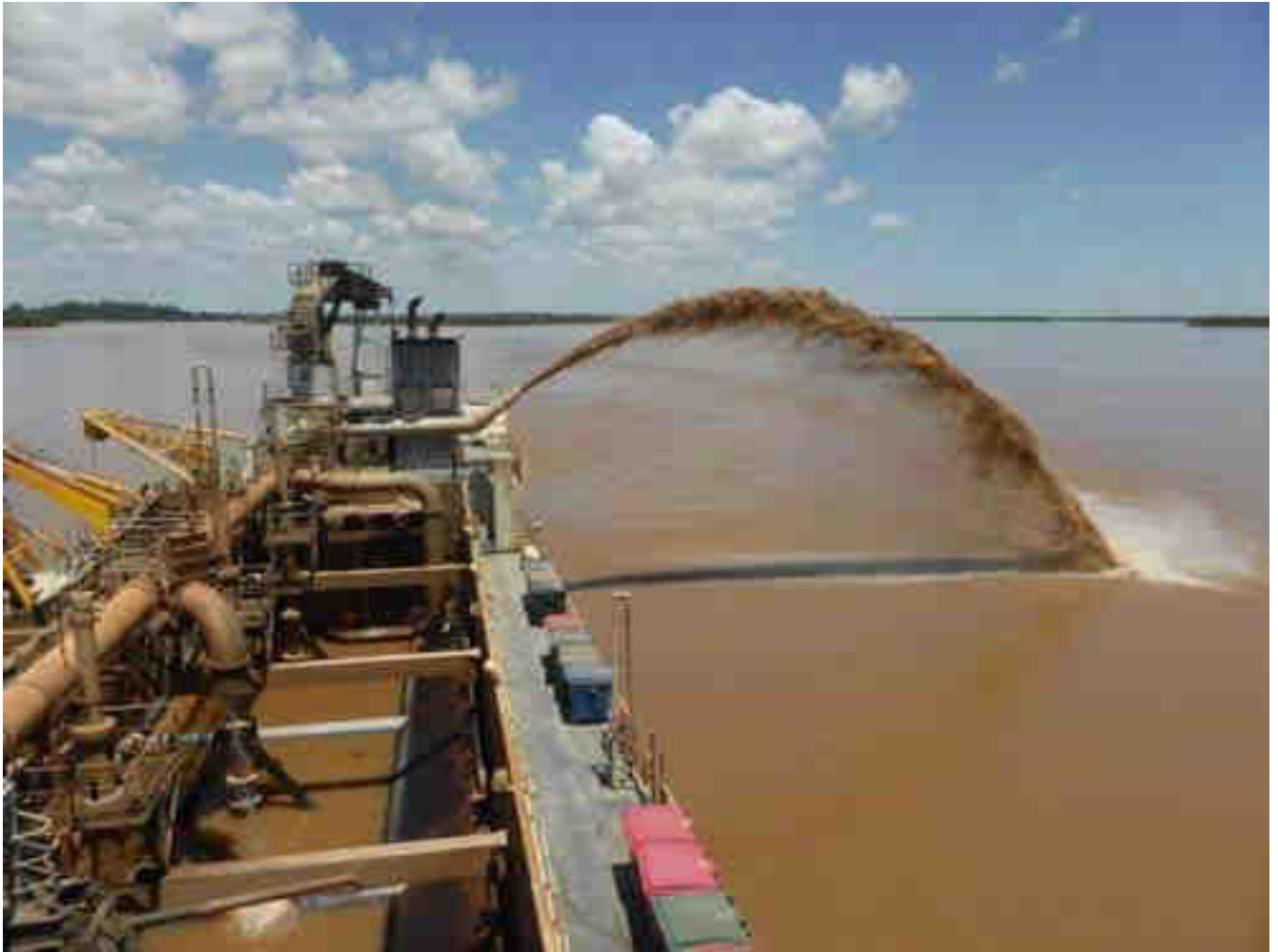
Figure 4-79: TSHD using sidecasting nozzle
