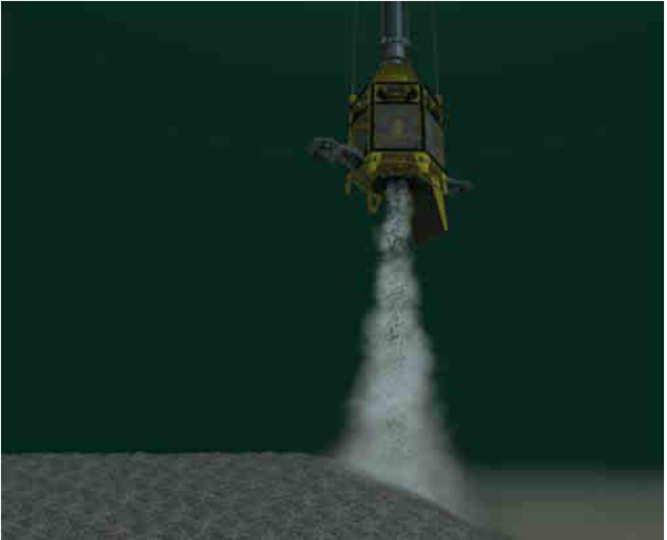
Figure 4-94: Rock installation via fall pipe with FPROV
