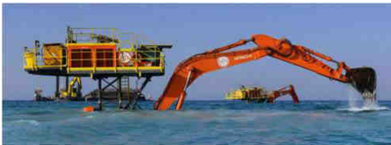
Figure 4-96: Starfish elevated excavator
