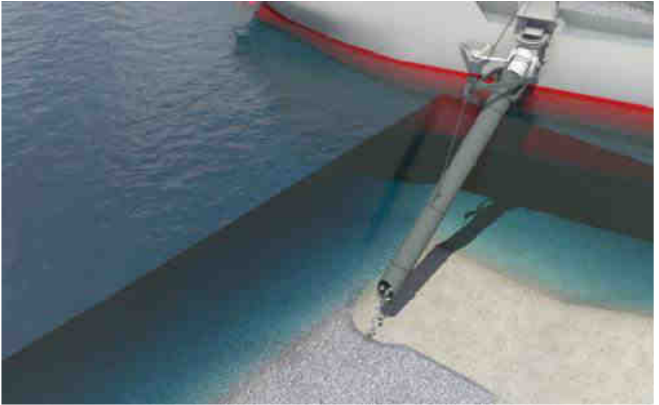
Figure 4-93: Rock installation with inclined fall pipe
