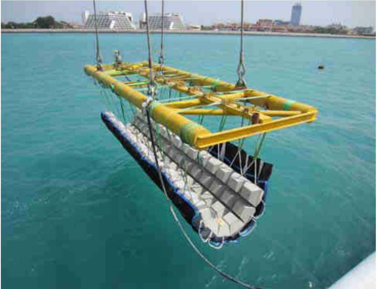
Figure 4-95: Example of concrete mattress for cable protection
