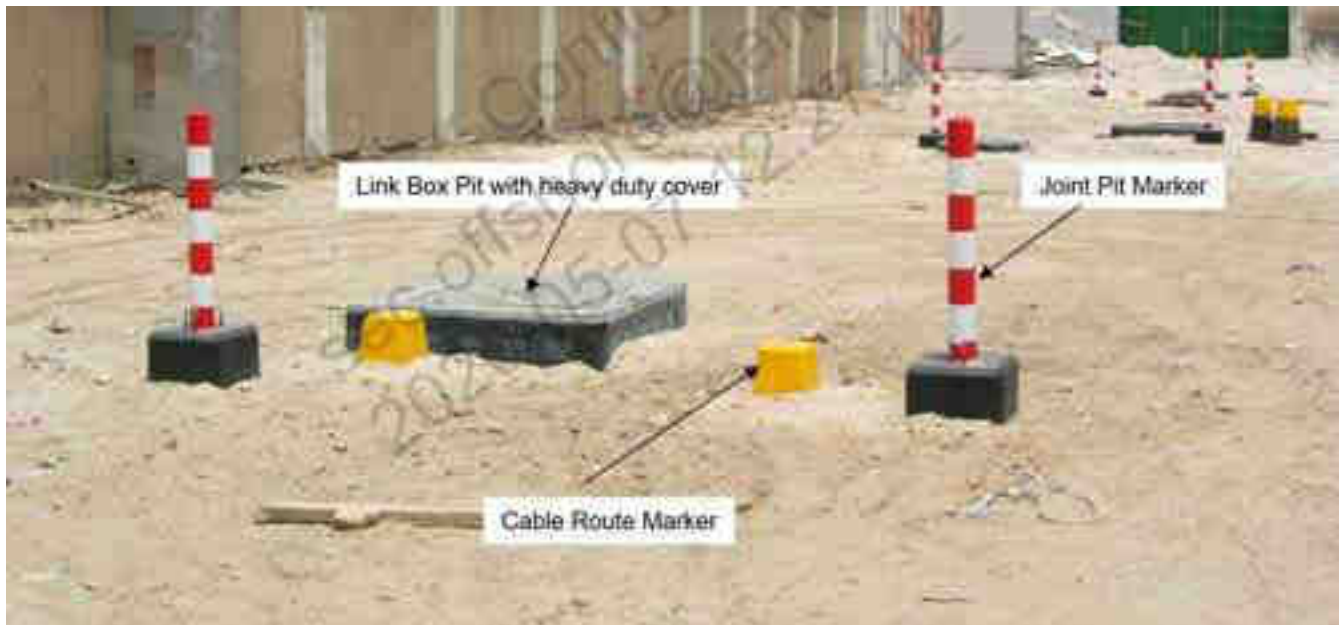
Figure 4-116: Example of TJB markers to be used at Shuweihat and Mirfa
