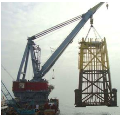
Levage de la structure ( www.heavyliftspecialist.com )
